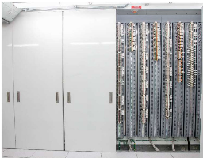
Figure 9 Sliding Doors on Marshalling Cabinets
