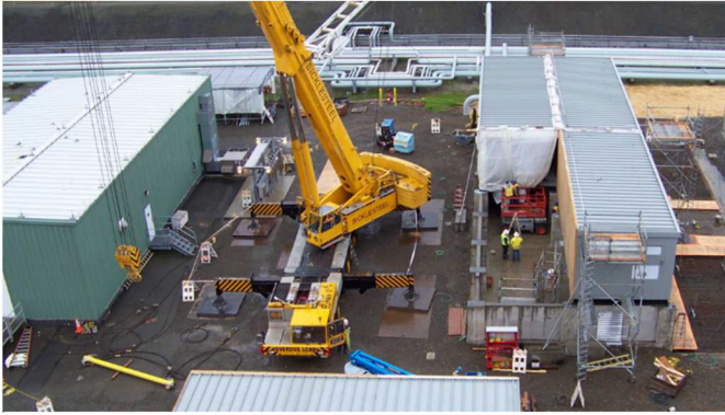
Figure 11 Assembly of A Prefabricated Substation
