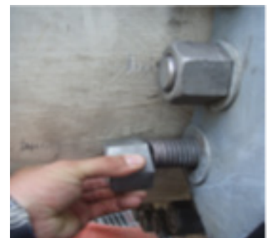
Fig. 6 FRP Flange/Nut Interference
